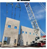
Using a simple three-step process—Set  $\rightarrow$  Place  $\rightarrow$  Tilt—IWS eliminates many of the costly and time-consuming steps of traditional installations. Because the windows are cast in place, there's no need for exterior caulking or finishing work at the frame-to-concrete interface. This eliminates common failure points and dramatically reduces long-term maintenance.
