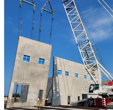
Using a simple three-step process—Set → Place → Tilt—IWS eliminates many of the costly and time-consuming steps of traditional installations. Because the windows are cast in place, there's no need for exterior caulking or finishing work at the frame-to-concrete interface. This eliminates common failure points and dramatically reduces long-term maintenance.
